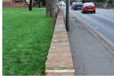
Church Litten Railings for Tanks
